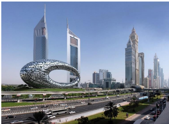
Picture 2: Affan Innovative Structures is making the façade of the Museum of the Future which is currently under construction in Dubai. The façade will be made of fiber-reinforced stainless steel. Copyright: Affan Innovative Structures.
