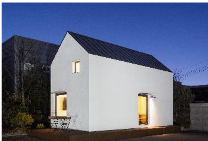
Picture 3: Pixel Haus® is AXIA’s new construction solution to build houses with composite sandwich panels. Due to the lightweight and size, it is possible to complete construction by simple assembly of the panels in less than a week still offering the same structural and finishing performance as conventional construction methods. Copyright: AXIA Materials.
